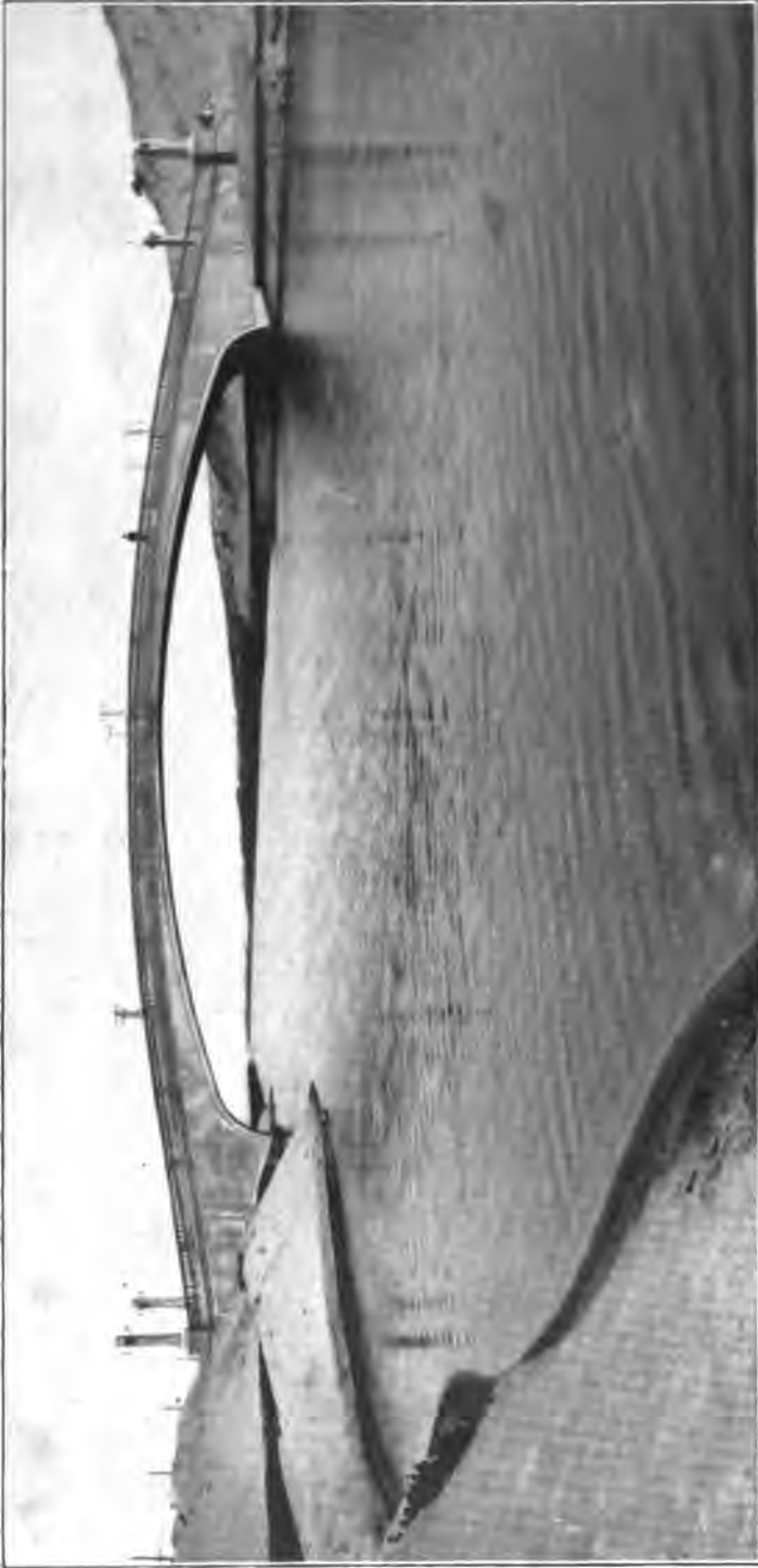
BRIDGE OF REINFORCED CONCRETE, AT PLAYA DEL REY, NEAR LOS ANGELES, CAL. Extreme Length, 265 feet 8 inches; Span, 146 feet; Width, 19 feet; Spring, 18 feet; Height above water, 20 feet.
